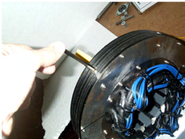
Mounting of the stator
